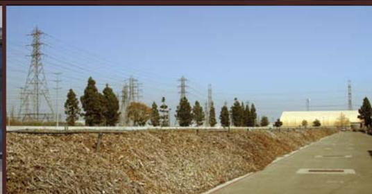
The biofilter contains over 50,000 cubic yards of chipped wood material piled onto a perforated floor. The facility exhaust air slowly travels through the 8-foot deep x 3-acre biofilter where odors and regulated compounds are removed.
