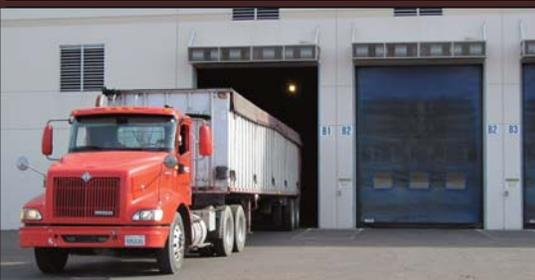
Trucks enter the building through high-speed roll up doors that close after each entry, preventing odors or dust from escaping.
