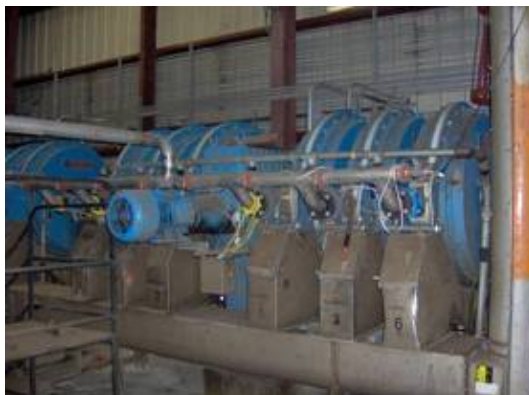
Figure 0-3 - Rotary Dewatering Presses and Sludge Conveyor
