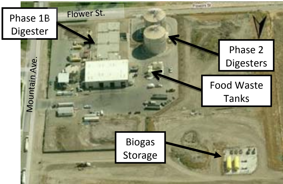
Figure 0-1 - RP-5 Solids Handling Facility
