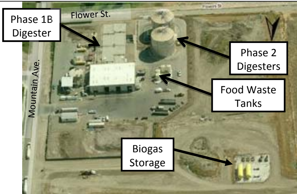
Figure 0-1 - RP-5 Solids Handling Facility
