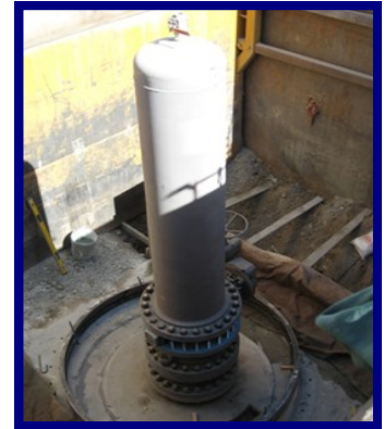
Valve installed at CB-14
