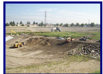
Construction of Berm No. 1 at Declez
