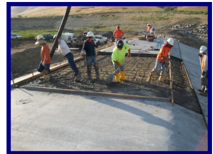
Construction Concrete Spillway at Declez
